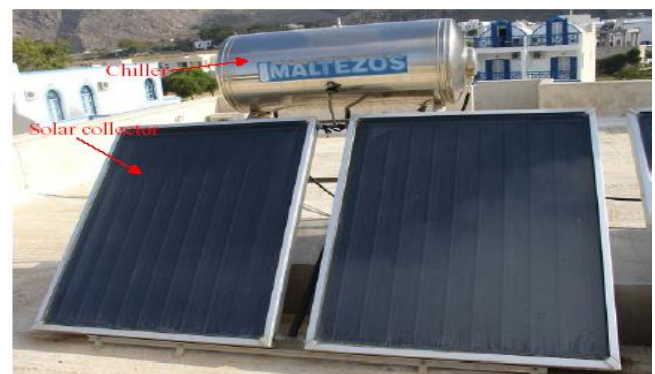
Fig: Flat-plate solar-powered single-effect absorption cooling system.
